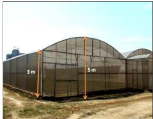
Permanent Insect proof net house in greenhouse design
