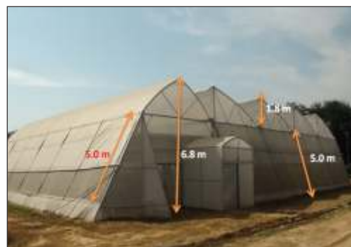
Multi-span Naturally Ventilated Green/Polyhouse
