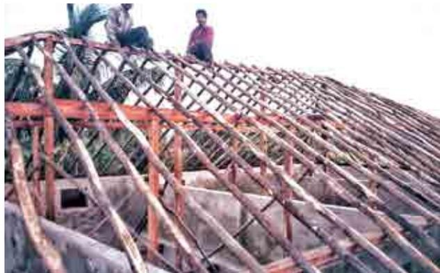
**Fig. 19.** Construction of housing units by utilizing self-grown raw materials at the farm
